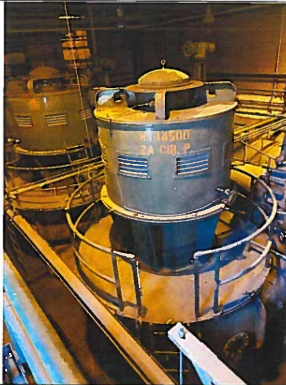
Photograph: 1 | Water Circulating Pump – Only 1 of 4 remains connected
